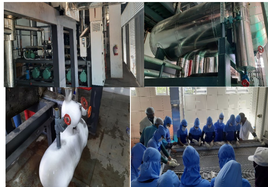
CO 2 -NH 3 cascade refrigeration system at NAS Fisheries Pvt. Ltd
