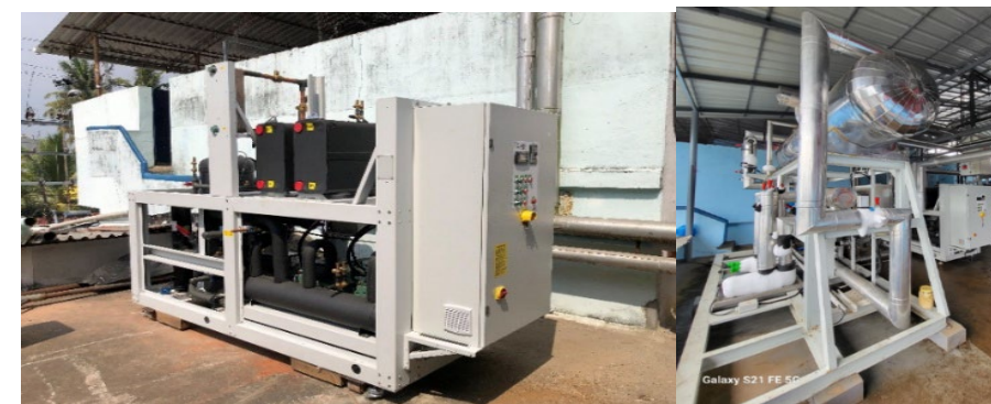
CO 2 -NH 3 cascade refrigeration system at Bellfoods Pvt. Ltd
